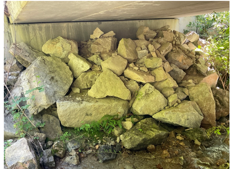
Left Bank Abutment when facing downstream
