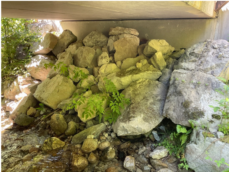
Right Bank Abutment when facing downstream
